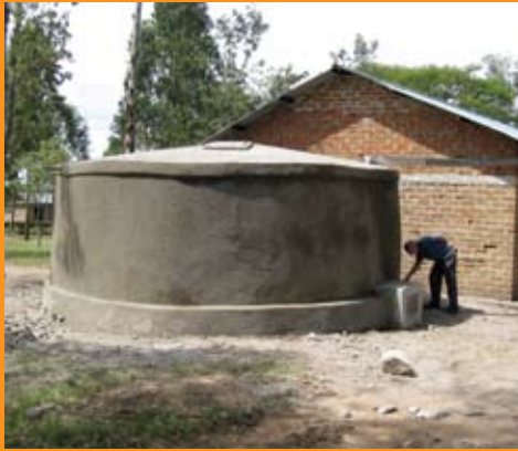
Kisangura Secondary – old cistern rebuilt (2009)
