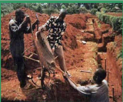
Davanga Village school – building the foundation
